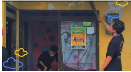
Figure 5. Activities cleaning up Ronda post before done painting wall.
