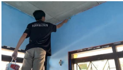
Figure 7. Painting process repeat wall corner read.
