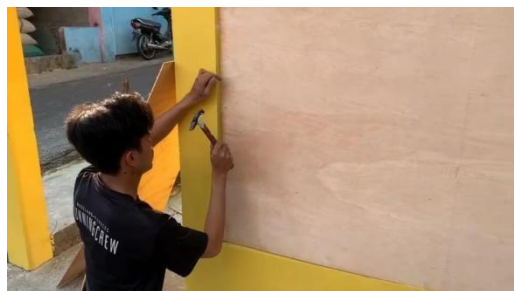
Figure 8. The installation process plywood For close glass existing window damaged
