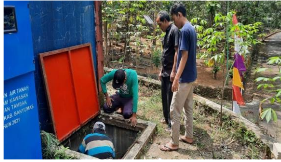
Figure 8. Checking and cleaning Brajageni water sources
