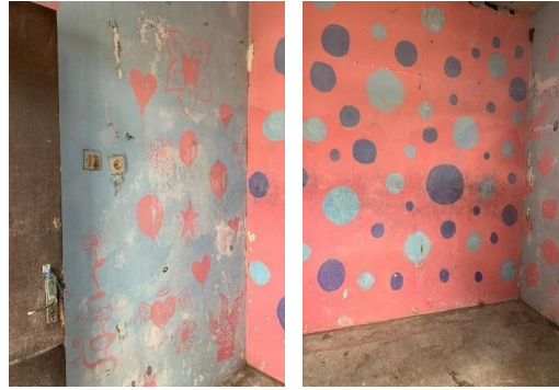
Figure 2. Wall view in Ronda office
