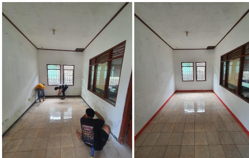
Figure 2. The room after being cleaned and in paint
